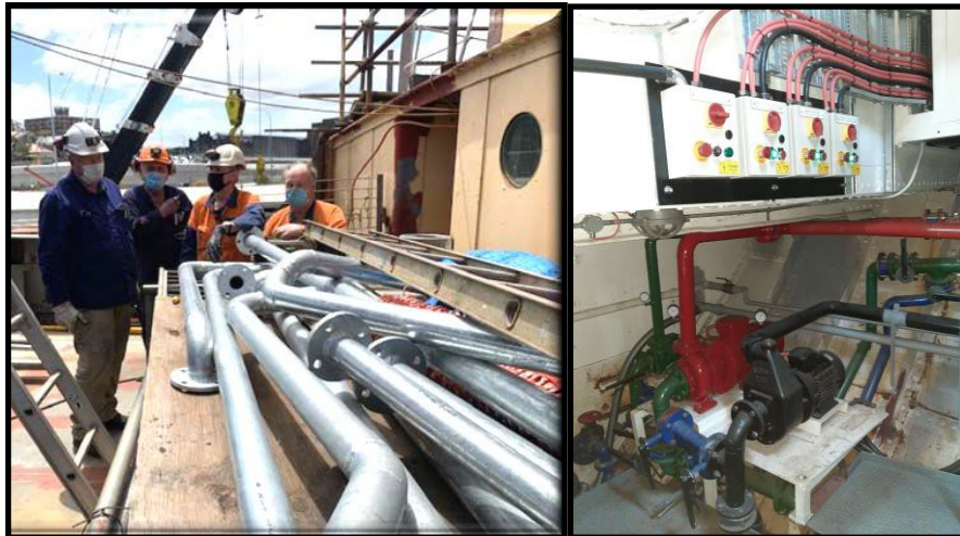
Bilge pipes just back from galvanising New pipessystems installed and painted
