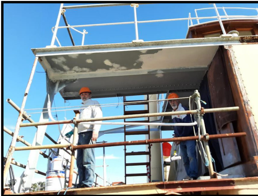
Cabin team applying coatings under Bridge Deck
