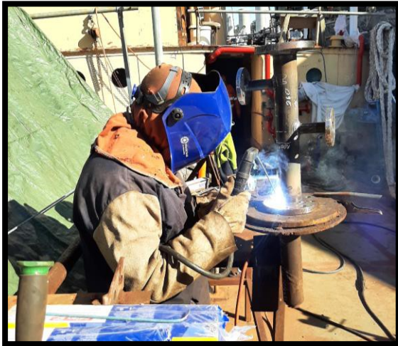
Welder Raj on steam pipe work
