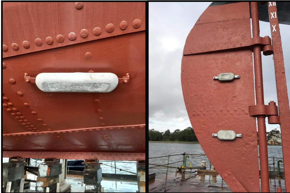
Hull anode installed
