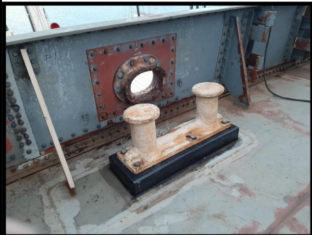
Well deck bollards set installed
