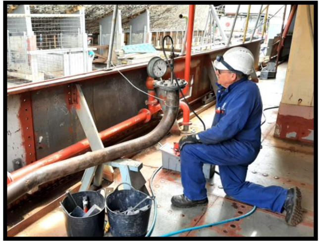
Engineer Malcolm pressure testing steam pipe
